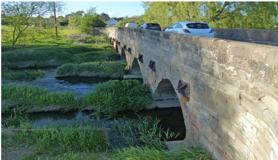
The Fosse Way Bridge over the River Avon in Bretford
